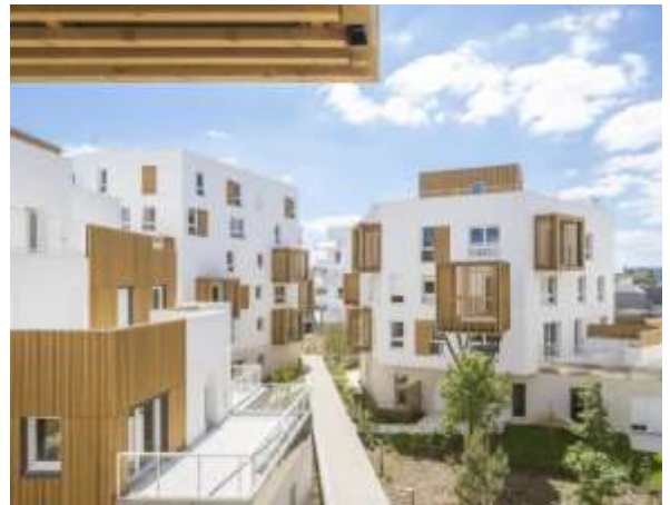
Residential complex in Romainville, architect Brenac Gonzalez, France, Paris.
