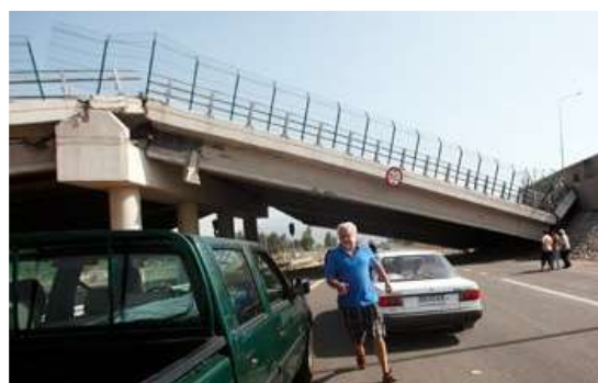
3 – rasm. Chili zilzilasi oqibatida yo‘lo‘tkazgichning buzilishi (2010 y.)
