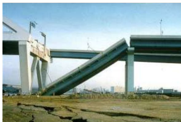
1 – rasm. Kobedagi zilzila vaqtida estakada oraliq qurilmasining qulashi (Yaponiya, 1995 y)
