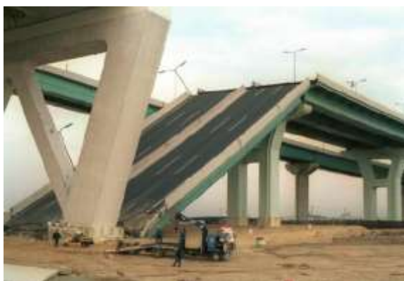
1 – rasm. Kobedagi zilzila vaqtida estakada oraliq qurilmasining qulashi (Yaponiya, 1995 y)
