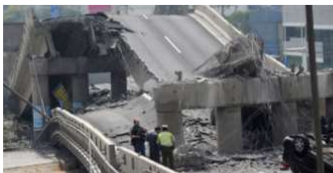
3 – rasm. Chili zilzilasi oqibatida yo‘lo‘tkazgichning buzilishi (2010 y.)
